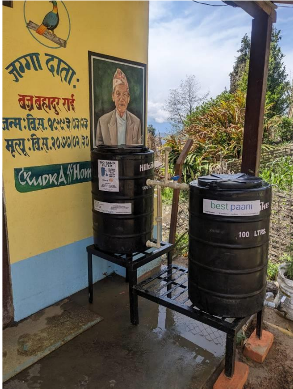
Figure 5: Installed Bio Sand Filters in School
